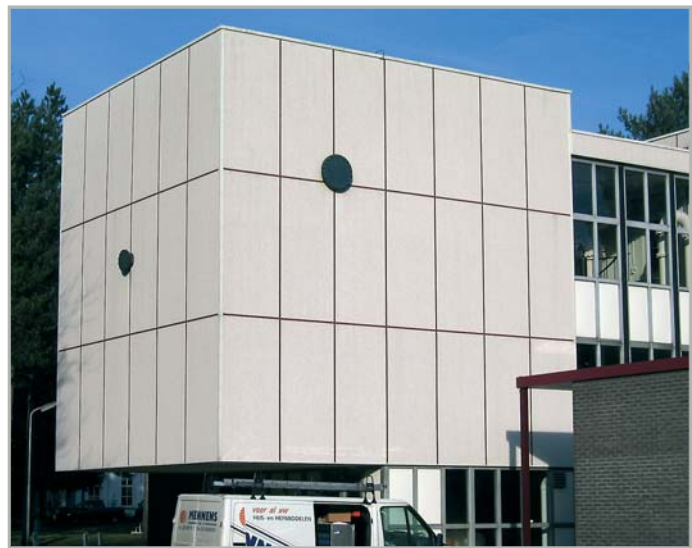
Concrete renovation in Laren, NL
