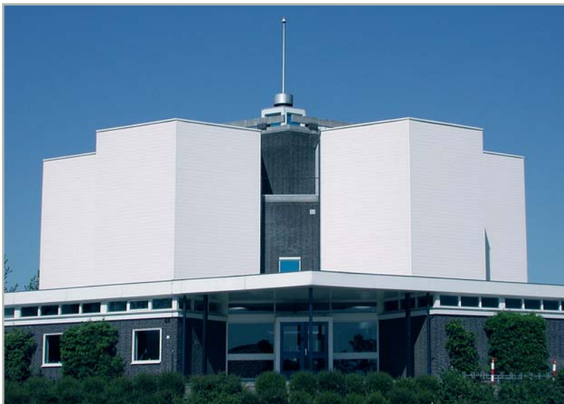
Water company building in Linschoten, NL
